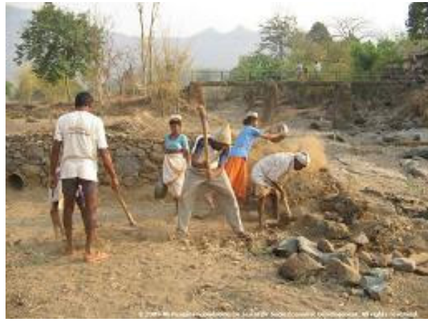
Figure 10: Work in progress at Dehrang
