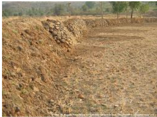
Figure 12: Damaged boundary has been fixed (Dehrang)
